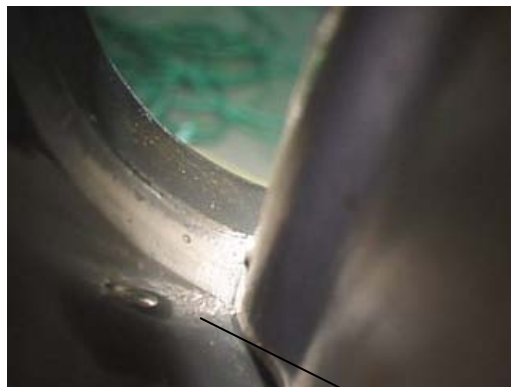
Note the worn area. This did not affect performance. Top Side
